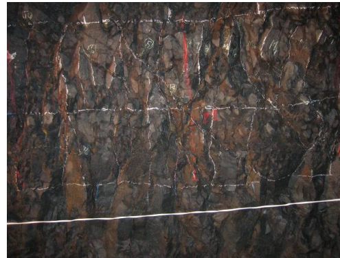
Fig.4 The Appearance of lower segment of weak weathering of Columnar Jointed Basalt(the 68 th adit in Baihetan dam site)
