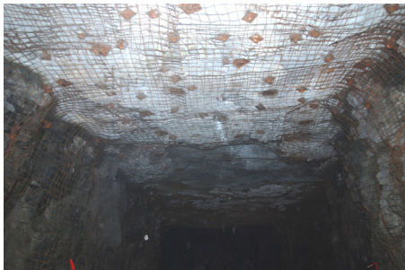
Figure 3. Reinforced backfill sill mat
