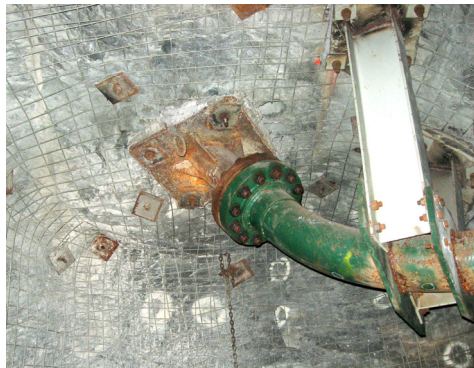
Figure 1. Reinforced borehole-to-level pipeline transition
