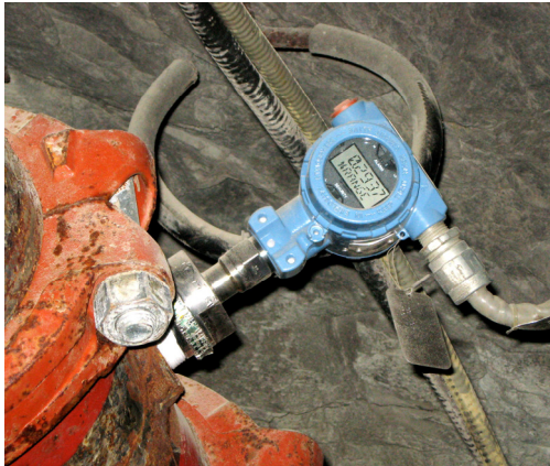
Figure 2. Backfill line pressure sensor
