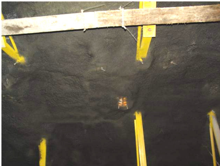
Figure 5. RockWeb applied to shotcrete over a winze sheave deck. Obstructions are easily sprayed around with little mess or overspray
