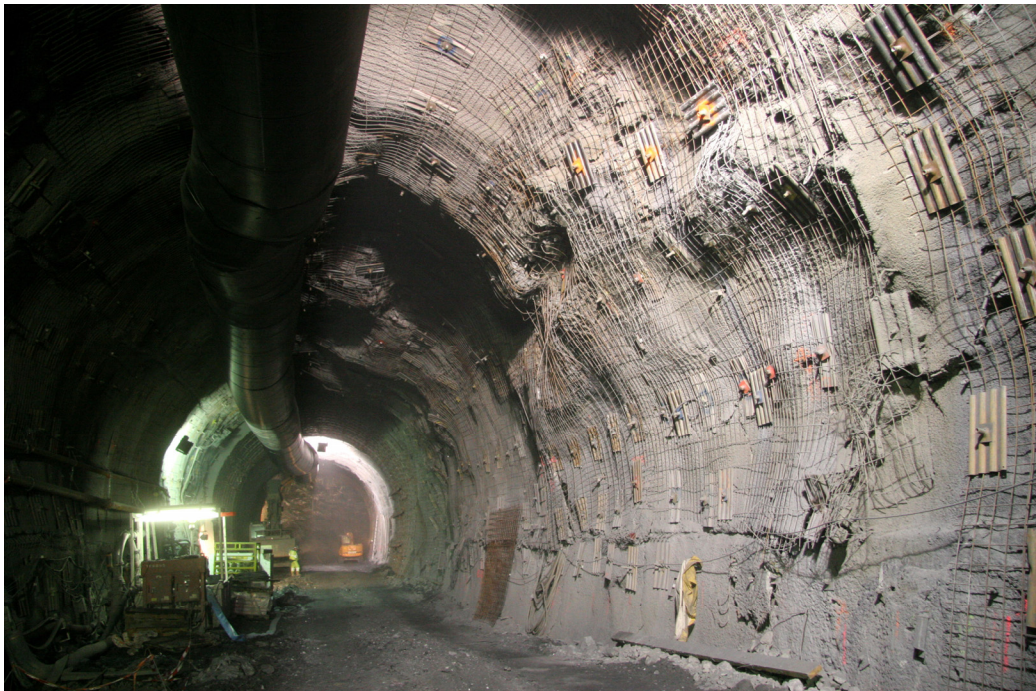
Figure 18. Deformations of the excavation contour of SMLP adit: see Figure 17 for comparison.
