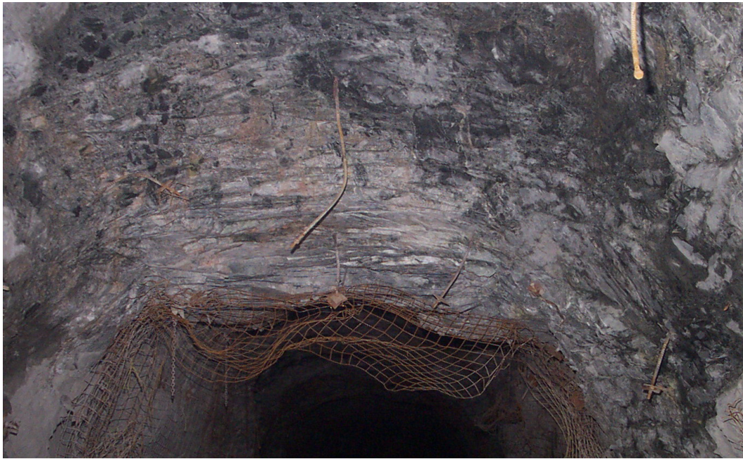
Figure 10. Evidence of stress-driven fracturing above excavation backs.
