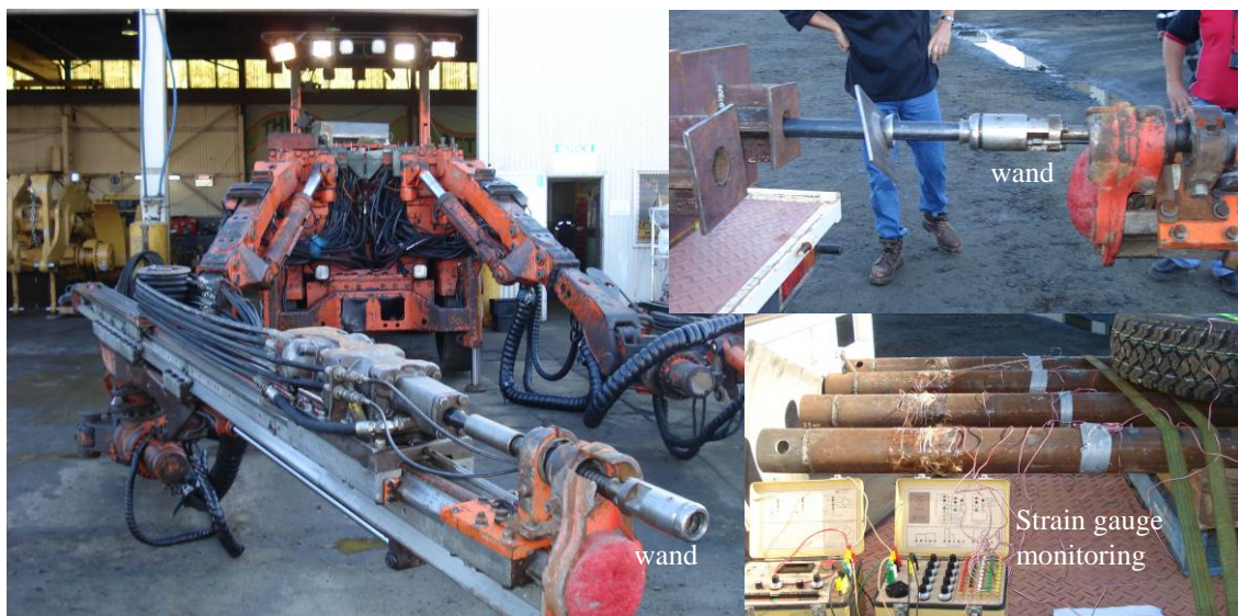
Figure 9. Omega bolt installation.
