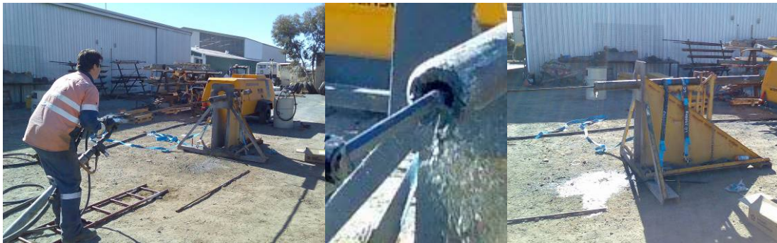
Figure 6. Airleg drilling of the sample to form the rough simulated borehole.
