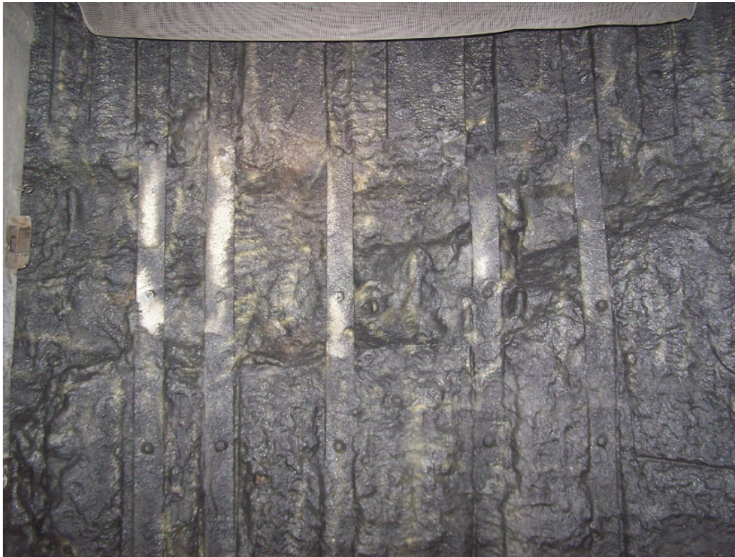
Figure 1. Steel straps and Rockweb spray-on liner installed to support the concrete wedge in the south wall of #3 Shaft.
