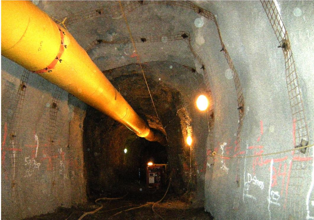
Figure 6: Enhanced support installed in burst prone areas
